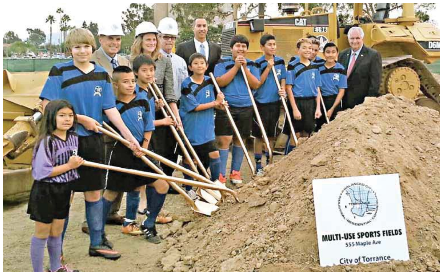
On Monday, Nov. 18, the City of Torrance broke ground on its new multi-use sports fields, located at 555 Maple Avenue. Mayor Frank Scotto announced the "kick-off of development." According to the City, more than 15,000 Torrance youth currently use City parks for sports practices and games, and the demand for field space is increasing. The new multi-use sports fields will also be used during the July 2014 AYSO National Games hosted in Torrance. Anticipated completion date is Feb. 2014. Pictured above are (L to R) L.A. Superior Court Asst. Supervising Judge Steven Van Sicklen, Former Assemblymember Betsy Butler, L.A. Superior Court Supervising Judge Mark Arnold, Field Deputy Representing the Office of Supervisor Don Knabe Steve Napolitano and Torrance Mayor Frank Scotto.
